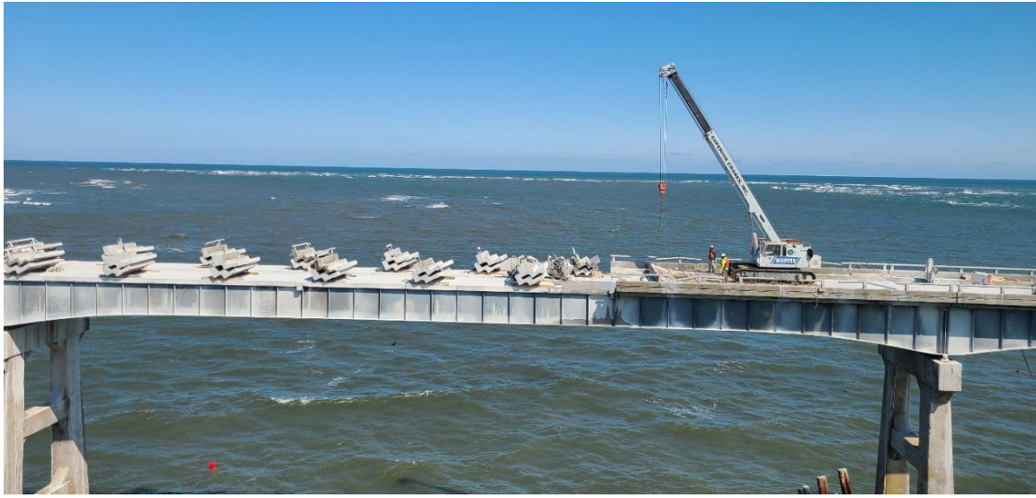
Figure 18 – Demolition of Span 145 (photographed on 3/5/2021 by NCDOT)
