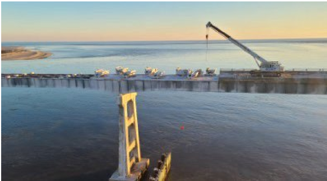
Figure 17 – Demolition of Span 145 (photographed on 3/4/2021 by NCDOT)
