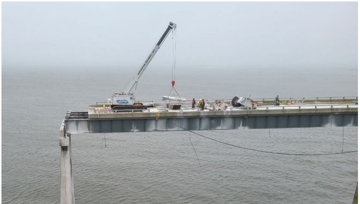
Figure 13 – Demolition of Span 144 (photographed on 2/15/2021 by NCDOT)
