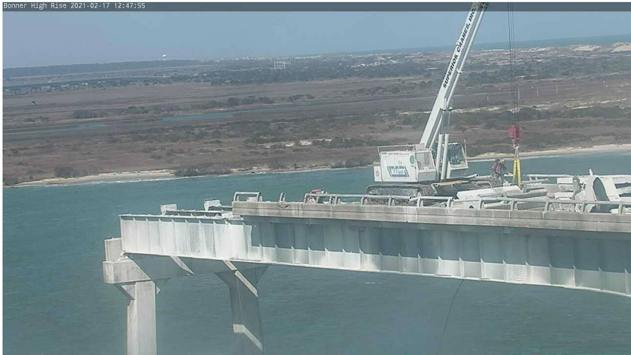
Figure 14 – Demolition of Span 144 (photographed on 2/17/2021 by NCDOT)
