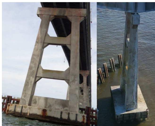
Figure 31 – Concrete deterioration
