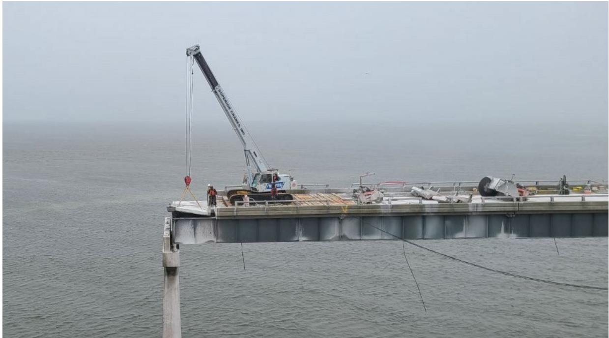
Figure 12 – Demolition of Span 144 (photographed on 2/15/2021 by NCDOT)
