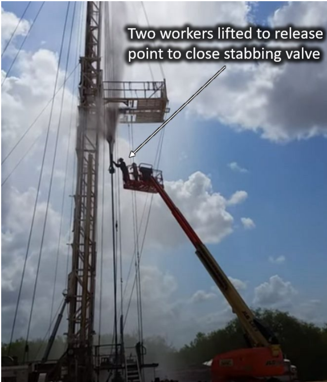
Figure 27. Two workers closing a stabbing valve following a blowout. (Credit: YouTube [27], annotation by CSB)
