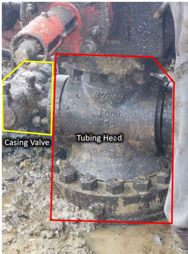
Figure 13. Existing tubing head with one of the casing valves attached. (Credit: Chesapeake, annotation by CSB)
