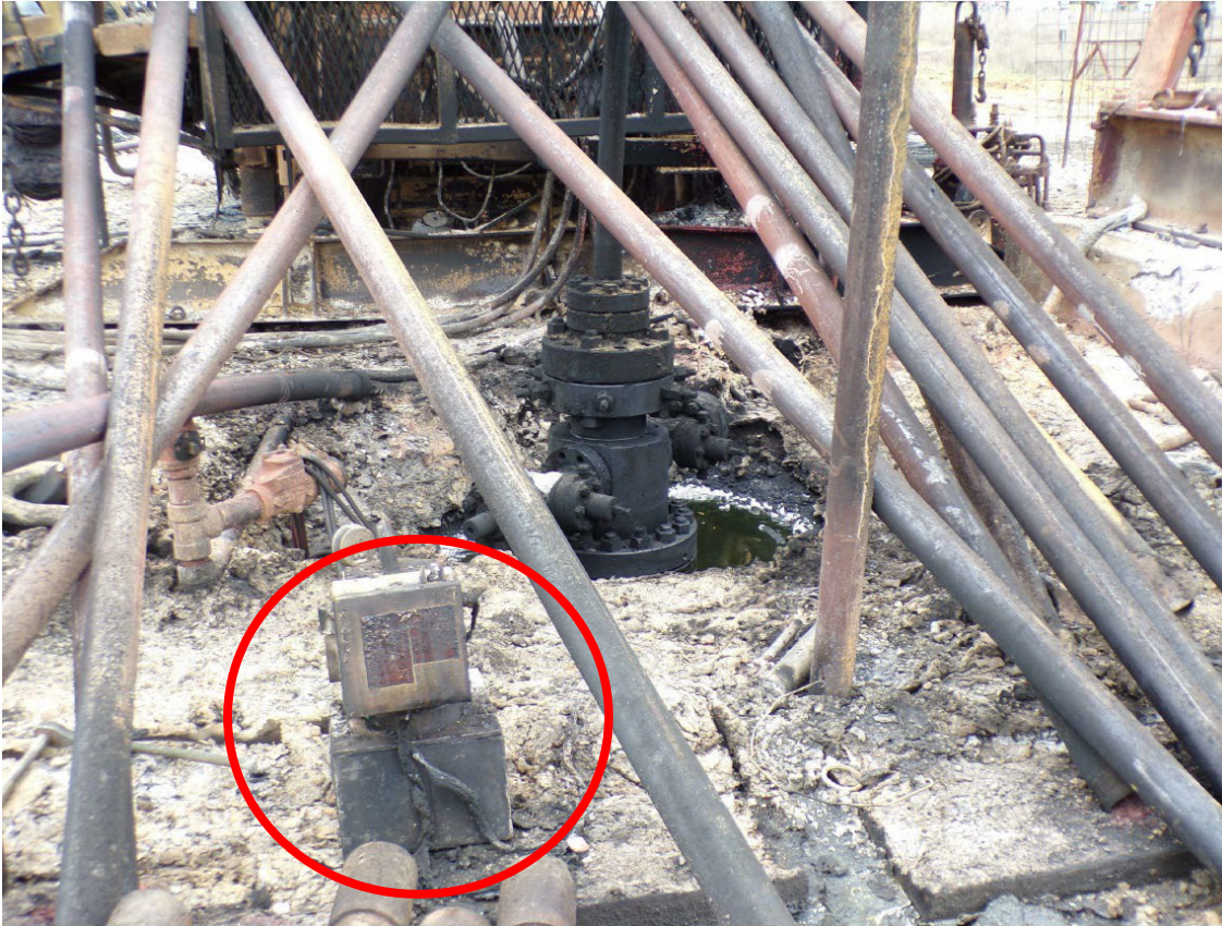
Figure 30. Hydraulic power pack (circled) location following the incident. (Credit: Chesapeake, annotation by CSB)
