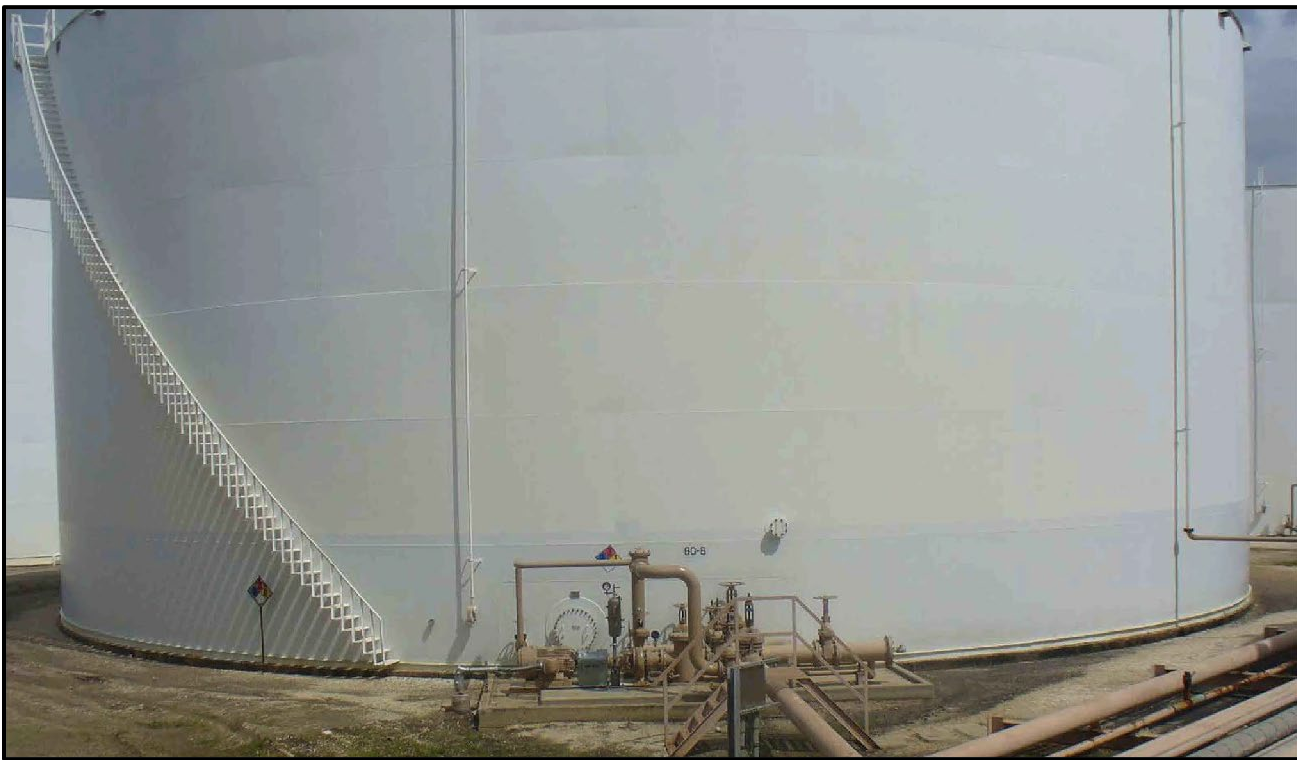
Figure 4. Tank 80-8, shown in 2007. (Credit: ITC)
