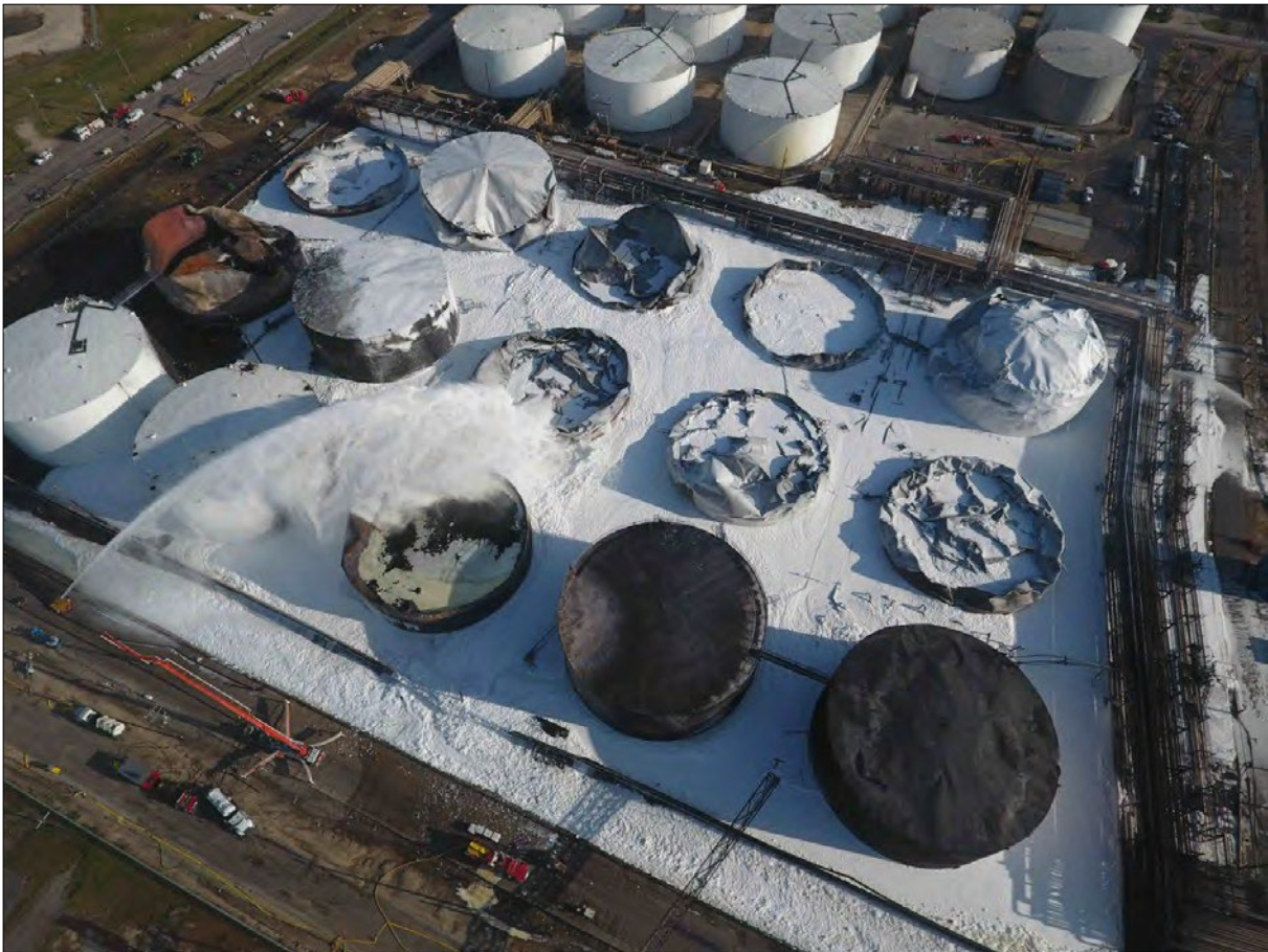
Tank Farm at the time of Containment Wall Failure, ITC First and Second 80's Tank Farm
