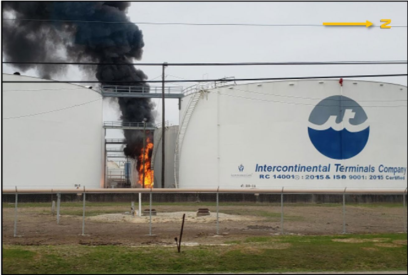
Figure 11. Initial ITC tank fire that ignited at Tank 80-8 on March 17, 2019. (Credit: HCFMO, annotations by CSB)
