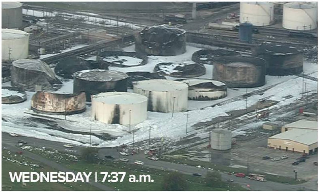
Figure 14. First & Second 80's tank farm on fire on Tuesday, March 19, 2019, and fully extinguished on Wednesday, March 20, 2019. (Credit: KHOU 11 News)
