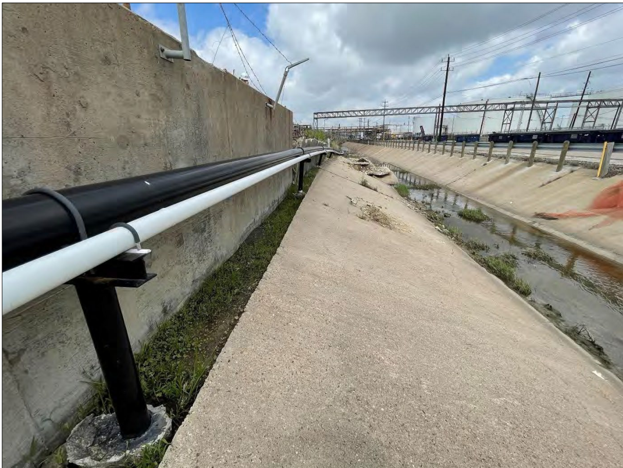
Photo 15: Drainage Ditch, undamaged section at north-east corner, looking west
