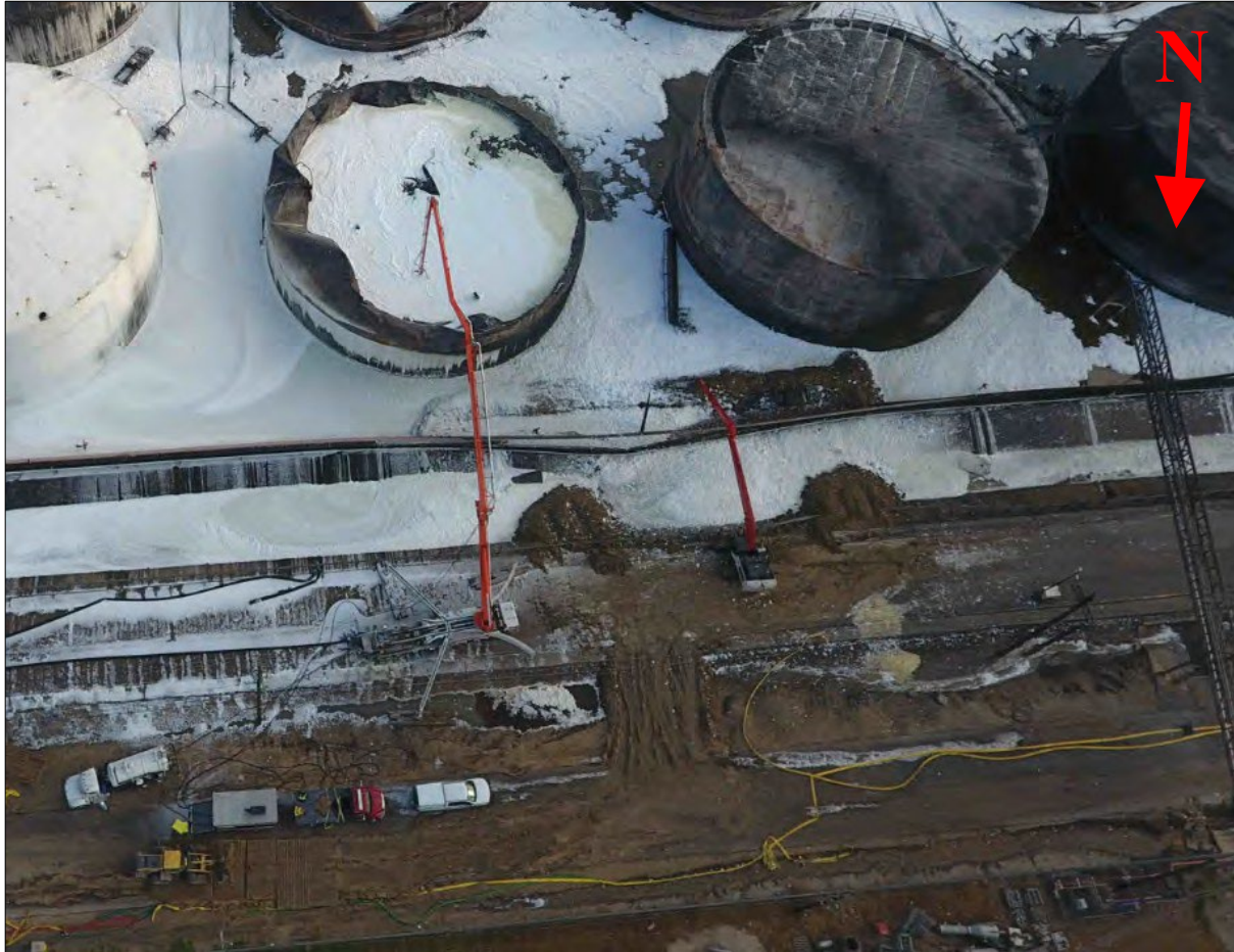
Photo 5: Responders constructing soil dike wall inside containment area to mitigate breach 13
