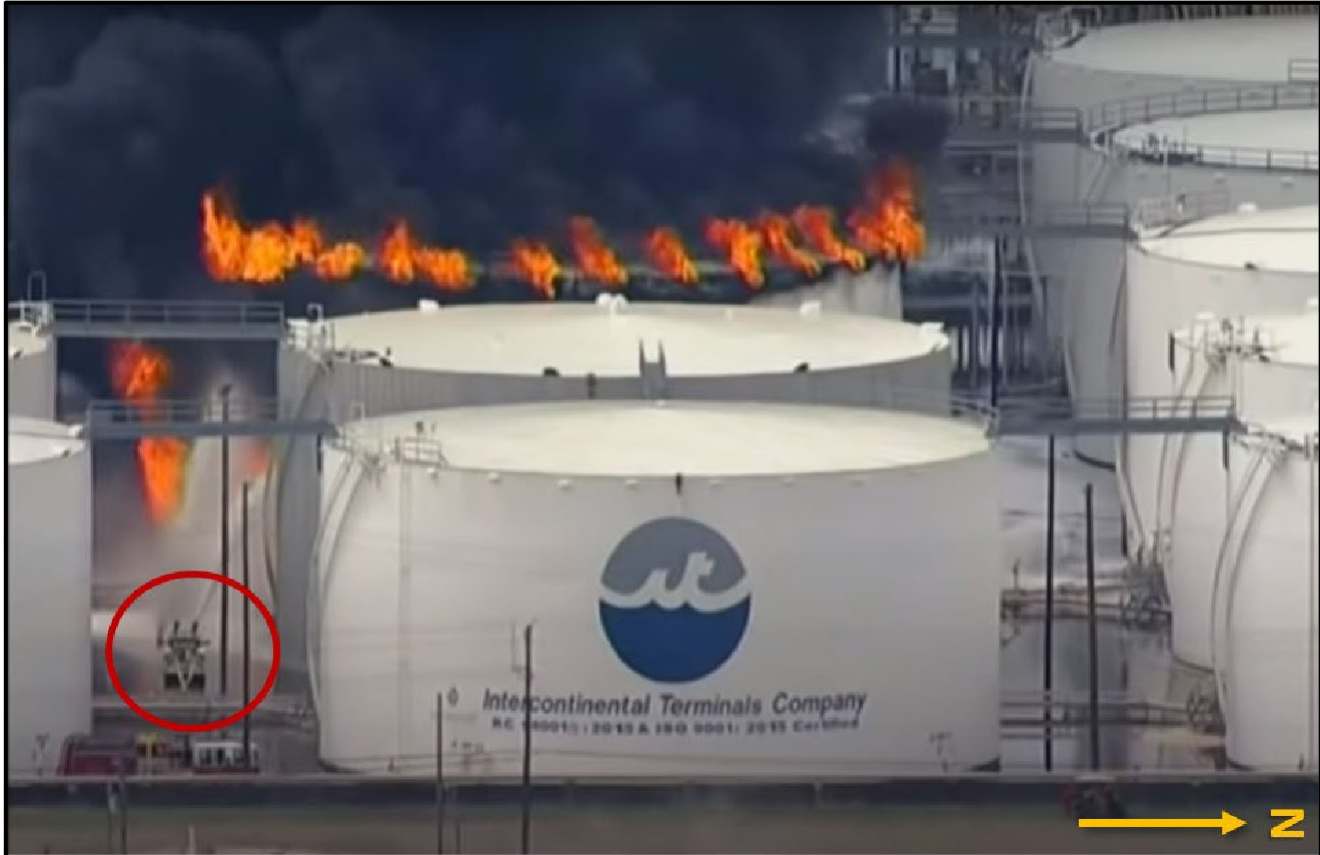
Figure 13. The quick attack truck (circled in red) staged between Tanks 80-11 and 80-12 on March 17, 2019. (Credit: Associated Press, annotations by CSB.)
