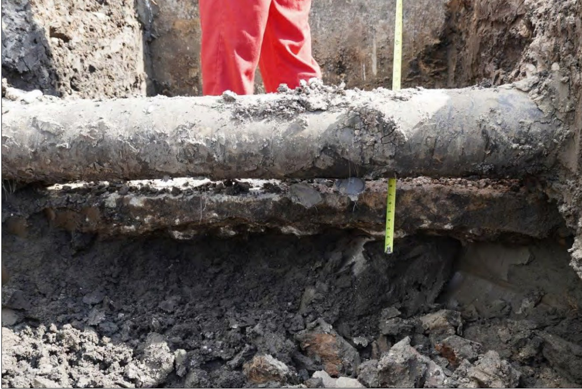
Photo 23: Containment wall footing and underside of footing
