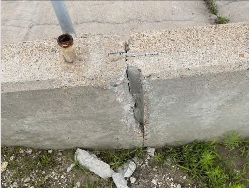
Photo 13: Construction joint with cast-in concrete shear key and centerbulb waterstop
