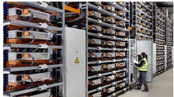
Figure 4.5: Second-Life Energy Storage Application for BMW Electric Vehicle Batteries
