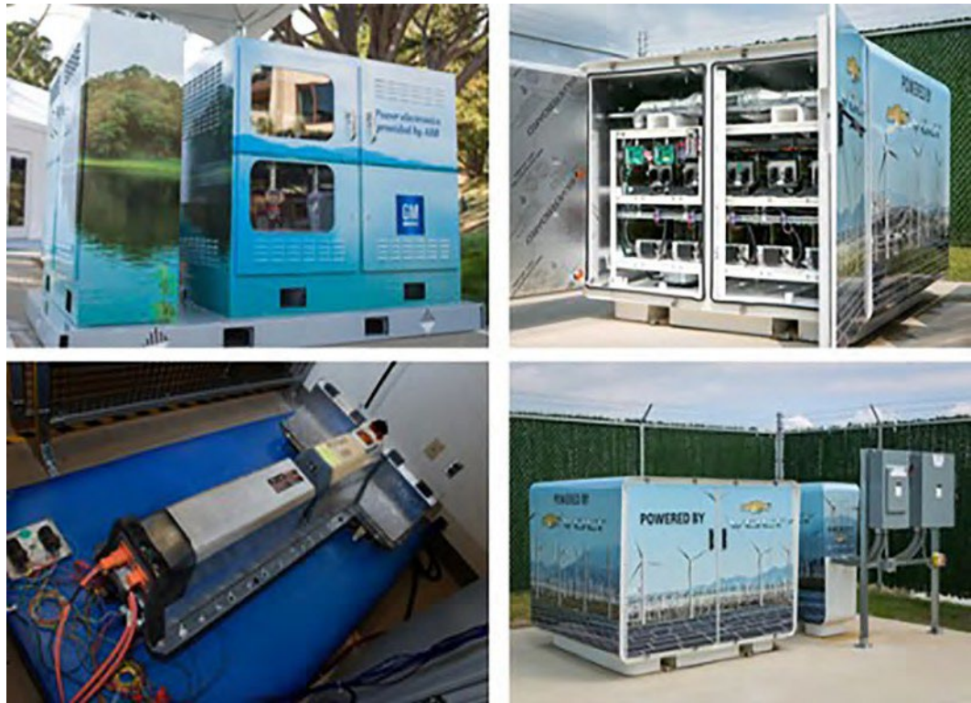
Figure 4.4: GM–ABB Second-Life Electric Vehicle Battery Applications
