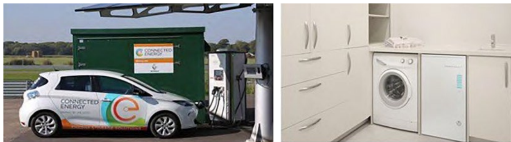
Figure 4.7: Renault–Powervault's Second-Life Electric Vehicle Battery Application
