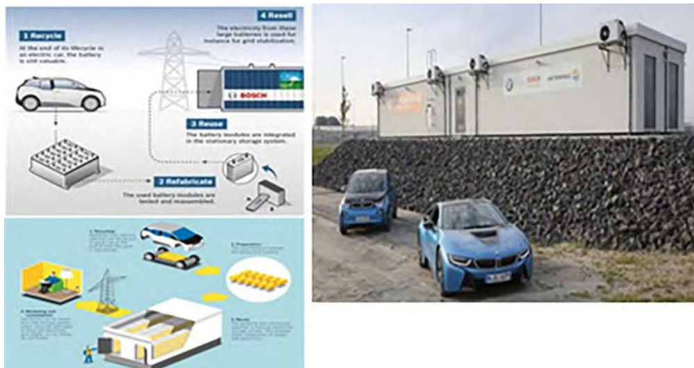
Figure 4.6: BMW–Bosch Second-Life Electric Vehicle Battery Demonstration Project
