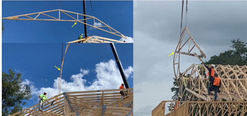
Figure 15 – Truss hoisting (Photo by WW Build)
