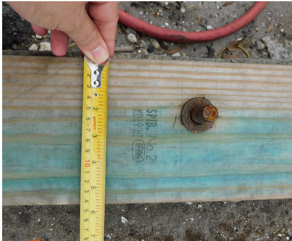
Figure 23 – Bearing wall frame – bottom plate
