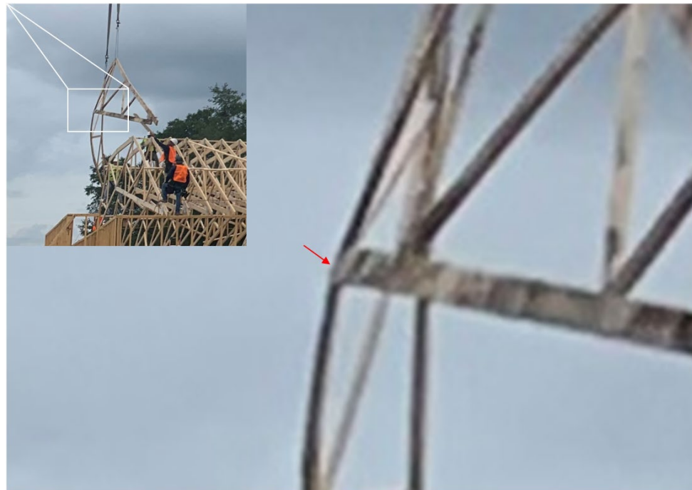
Figure 16 – Truss hoisting (Photo by WW Build)
