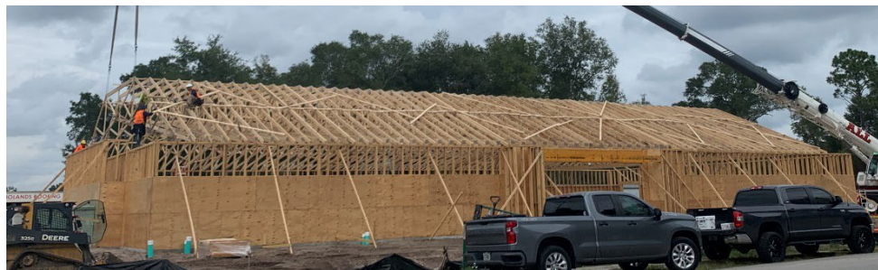
Figure 5 – Bearing walls and trusses – looking north (Courtesy of WW Build)
