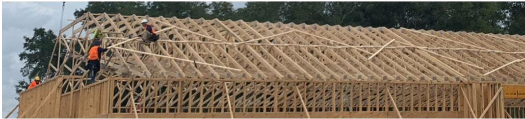
Figure 12 – Truss braces at the south side – looking north (Photo by WW Build)
