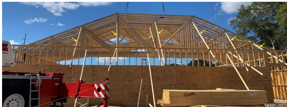
Figure 8 – Truss diagonal end braces at the east side – looking west (Photo by WW Build)
