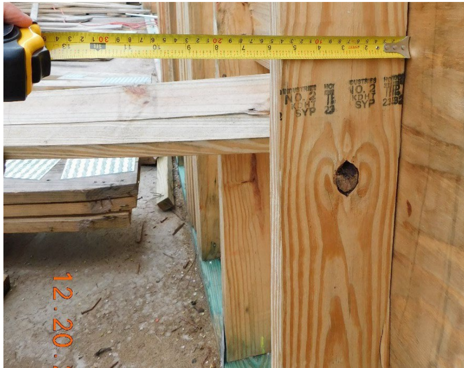
Figure 21 – Bearing wall frame – studs
