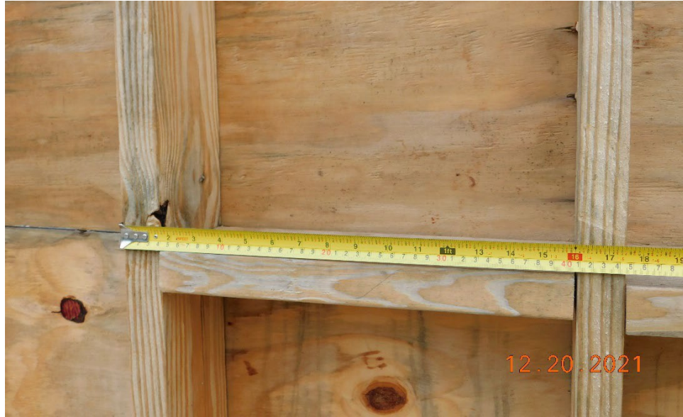
Figure 22 – Bearing wall frame – studs
