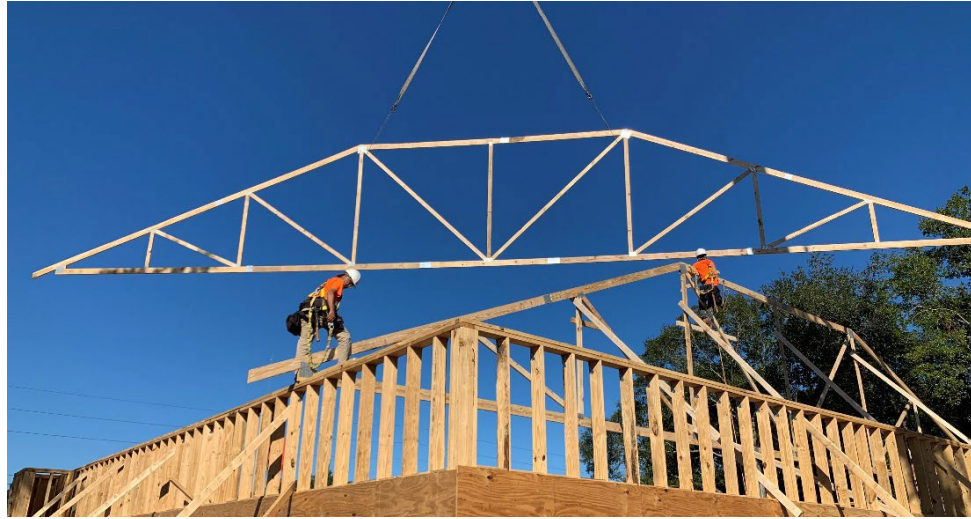
Figure 7 – Truss erection – looking northwest (Courtesy of WW Build)
