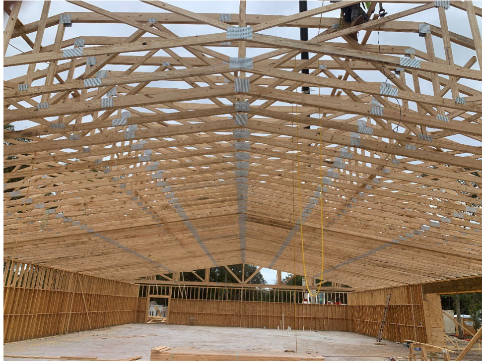
Figure 14 – Truss bottom chord – looking east (Photo by WW Build)
