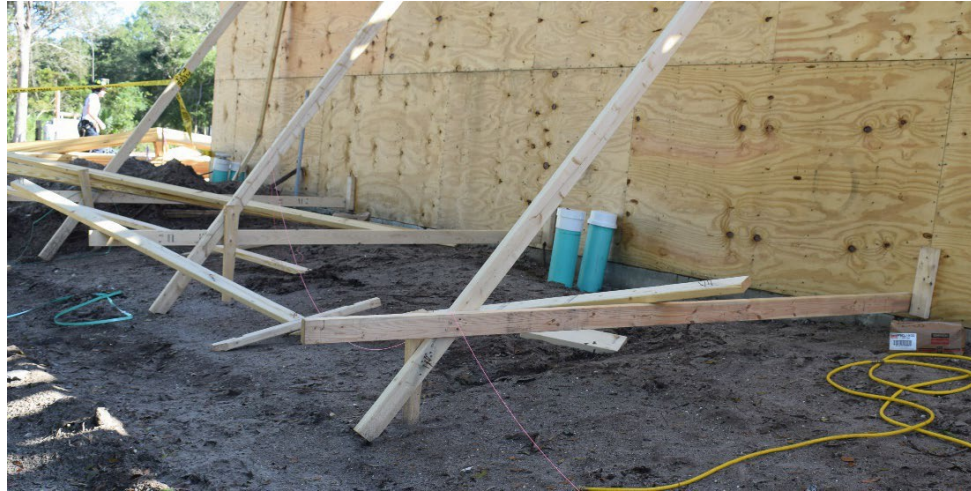
Figure 24 – Bearing wall frame – diagonal bracing
