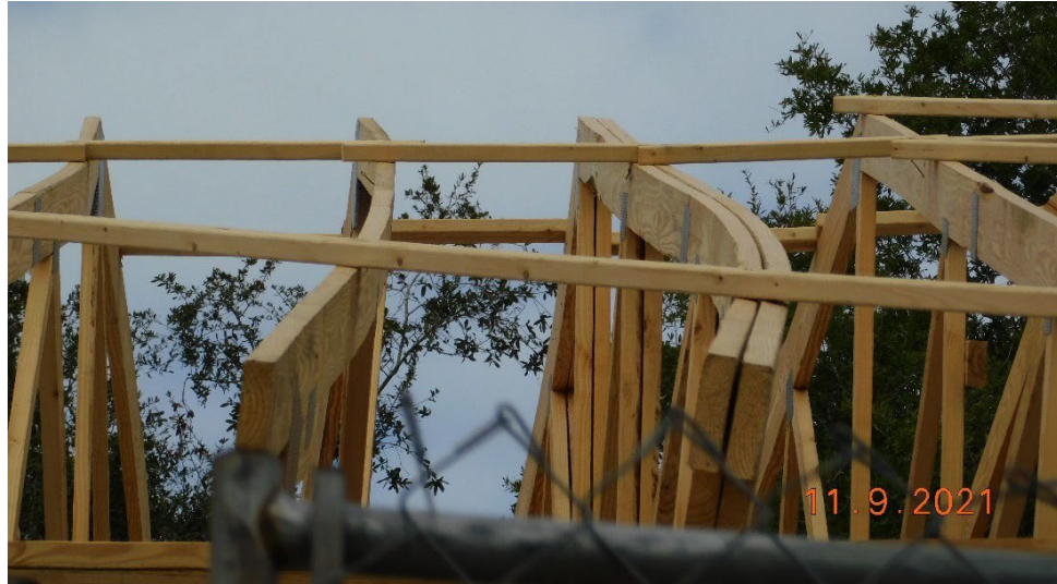
Figure 17 – Buckled trusses
