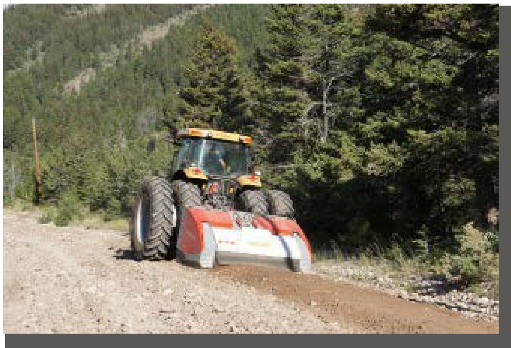
An example of a tractor-mounted crusher processing coarse material in-place.
