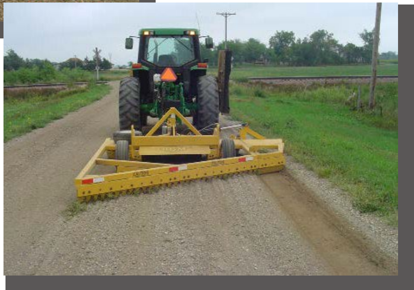
Example of a light blading device being towed by a mower tractor.
