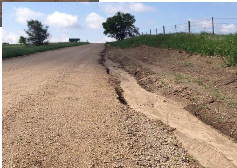
This road is located in mountainous terrain, yet the motor grader operator has been able to maintain a small ditch for roadside drainage and the road performs well.
