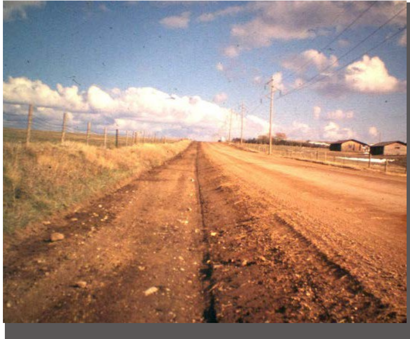
Excellent roadway reshape done with only motor graders, a roller and water truck.
