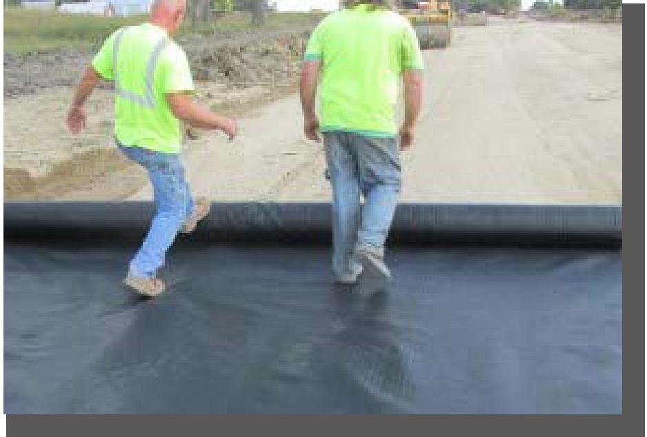
Good example of rolling fabric out over well prepared subgrade.
