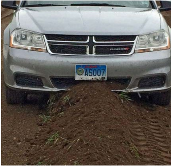
Berm too large for motorists to traverse. (Source: Bruce Drewes, 3T Group LLC).
