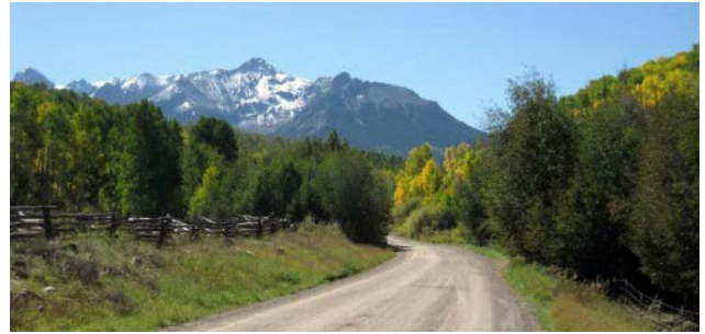
Example unpaved road owned by the U.S. Forest Service (Source: Unpaved Roads Less Traveled Blog).
