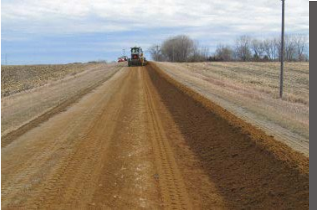
This operator had done an excellent job of completely windrowing and equalizing the new gravel . . . .
