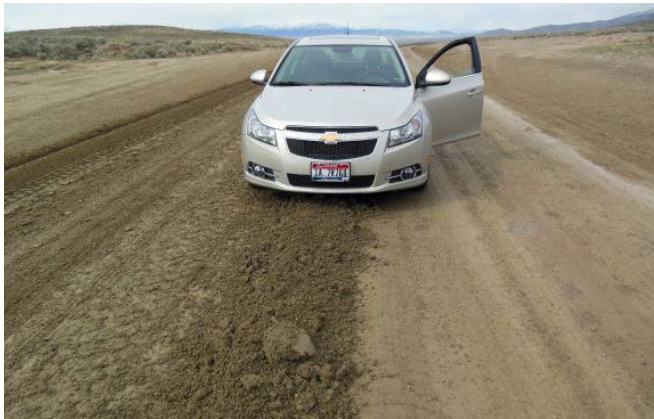
A small berm presents lower risk to the motorist. (Source: Bruce Drewes, 3T Group LLC).
