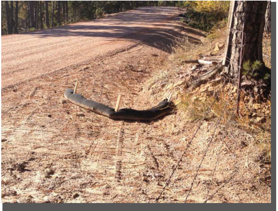
Good example of basic erosion control after gravel road reshape.
