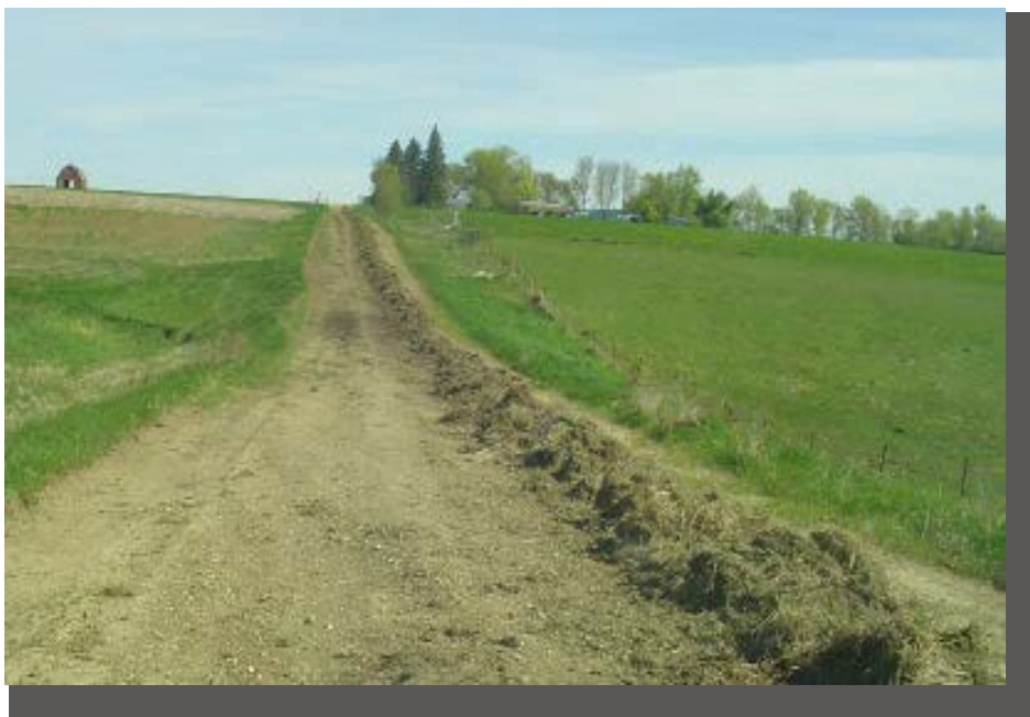
This windrow is excessive and should never be left on the roadway. It is a bad practice even on a very low volume road. Multiple passes should have been made with the grader to work the vegetation out of the windrow or other mechanical means such as a disk should have been used to break up the chunks of sod so more material could be spread on the roadway.
