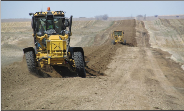
Reconstruction work space. (Source: Greg Vavra, SDLTAP).
