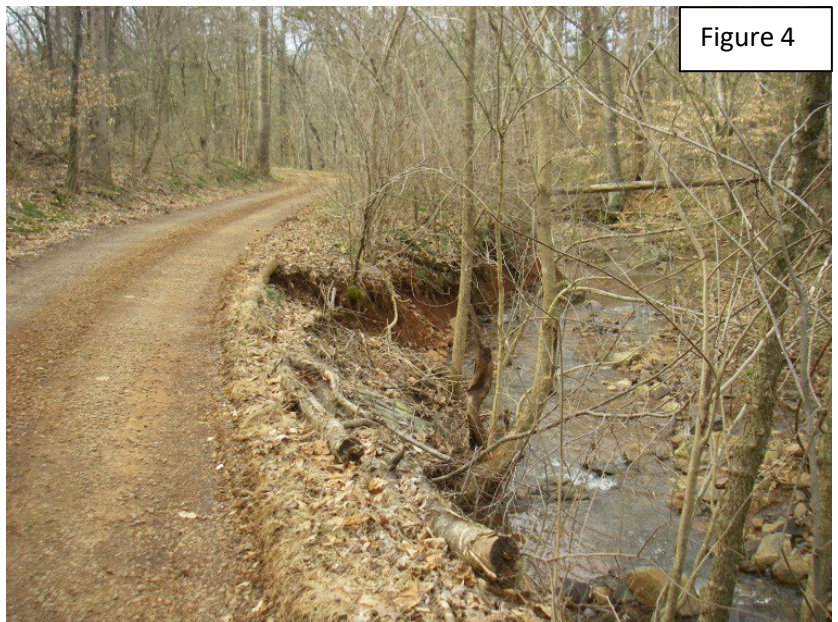
Figure 4: A road that follows close to the stream will erode.
