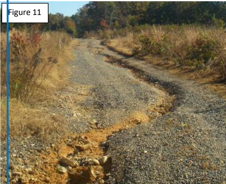
Figure 11: Lateral erosion across the roadbed, see #2.
