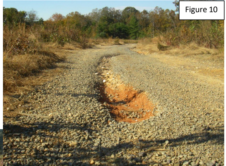
Figure 10: Erosion down the roadbed, see #1.
