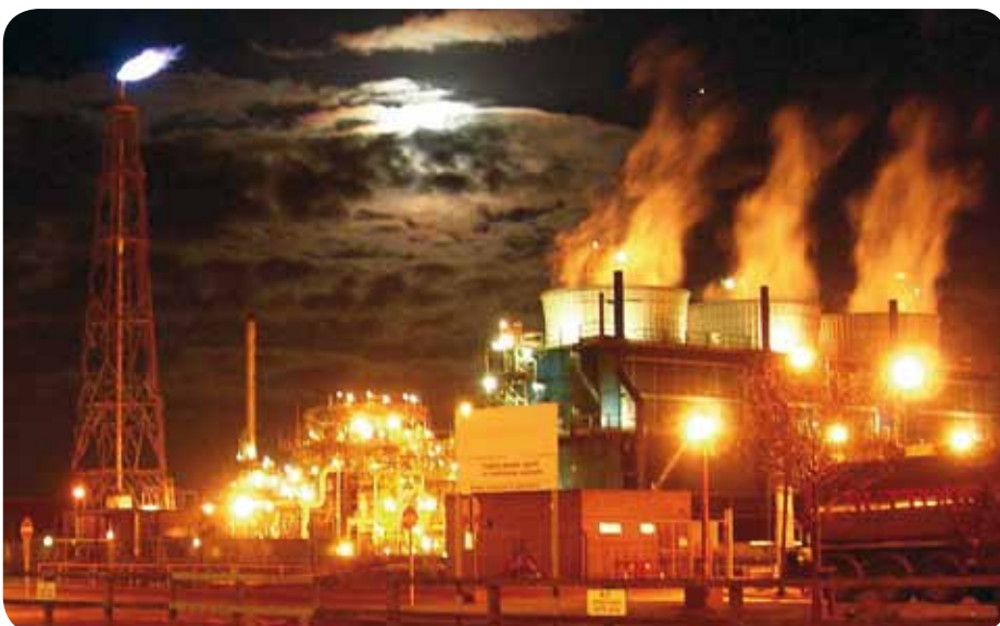
Fig. 4.7: Energy intensive industries are responsible for about 10 GtCO 2 -emissions (10 000 million tons of CO 2 per year) through using about 37 percent of global energy. The contribution of renewables to this already highly energy-efficient sector is – and will stay – low.
