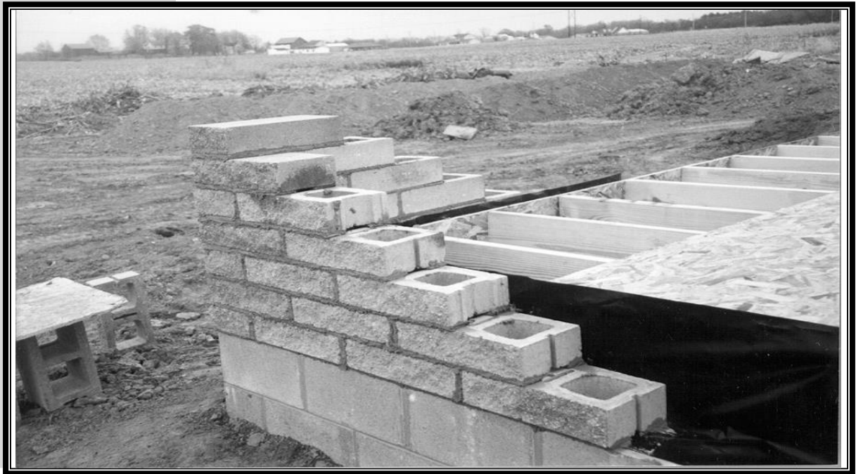
FIGURE 1.6 House Construction Using Concrete Masonry
